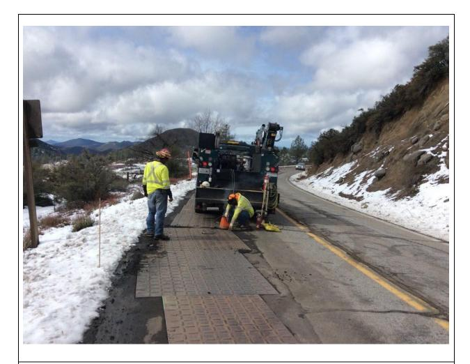
**Photo 4:** In accordance with the CFPPP Fire Matrix for hot work on CNF land with a PAL A, a Designated Fire Patrol was present and a full set of fire tools was observed within 50 feet during welding along Sunrise Highway (C 440).
