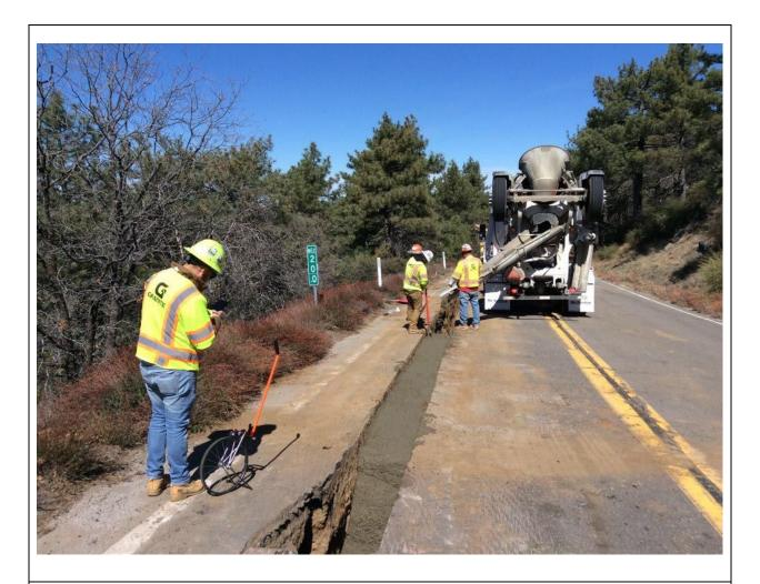
**Photo 2:** Crews were observed slurrying in the conduit package along Sunrise Highway (C 440). Crew members were observed displaying hard hat stickers indicating that they had completed project WEAP training in accordance with MM BIO-2.
