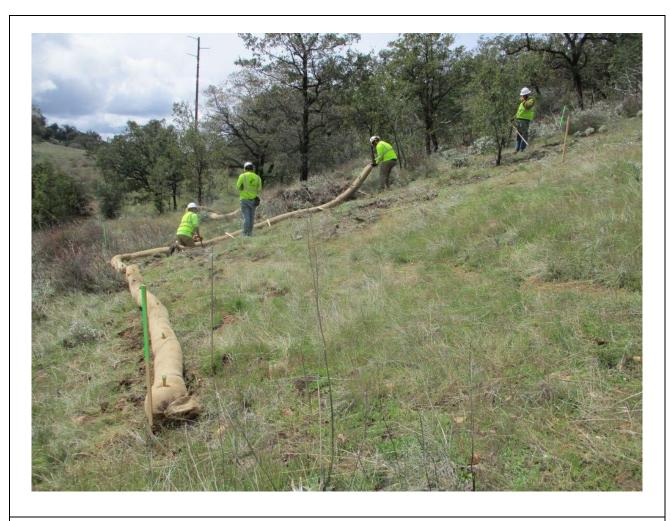
**Photo 6:** A crew was observed installing erosion control BMPs at Pole P259364 (TL 626 Conversion North) in accordance with the ECP and SWPPP.
