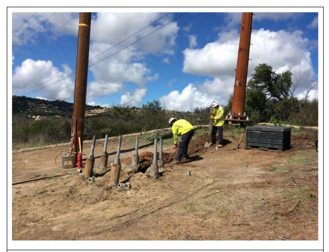
**Photo 1:** During ground rod trenching at Pole Z105011 (TL 6923), a full set of fire tools (5-gallon backpack pump, round point shovel, Pulaski, and 2A10BC fire extinguisher) was observed within 50 feet of the activity in accordance with the CFPPP.
